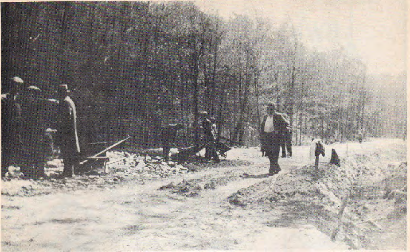
Shovels and wheelbarrows were the main tools used during the construction of Highway 35. This photo, showing a stretch of the highway work near Halls Lake, was taken in 1934. (Photo courtesy of Ethel Greene)
